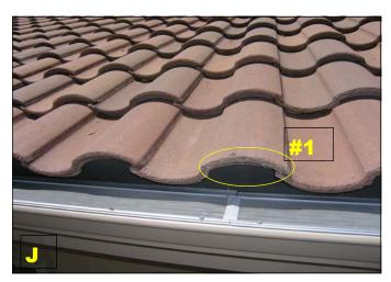
8. **VERY IMPORTANT!** On these types of roofs where there are large upward corrugations (see #1 in **Photo J** above) the finger fastener MUST go under the upward corrugation. If you put the finger fastener on the lower corrugation, so much water comes down that it may run off the finger!
