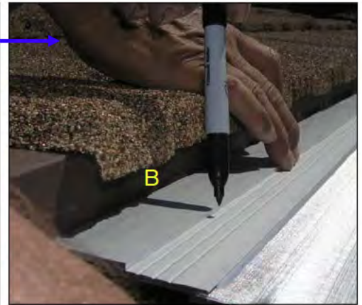
Figure A: The one inch strip fits neatly on top of Gutterglove covering the gap between the fascia board.
